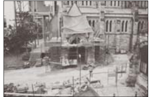
1989 Construction of the West End begins with the South West Porch.
