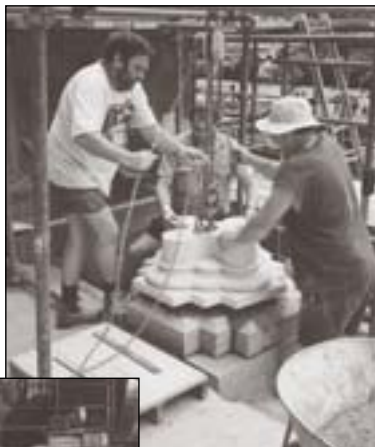
Stone masons Allan Kerr, Cliff Lawrance, foreman, and Dave Pocock laying a column base in the West End.
