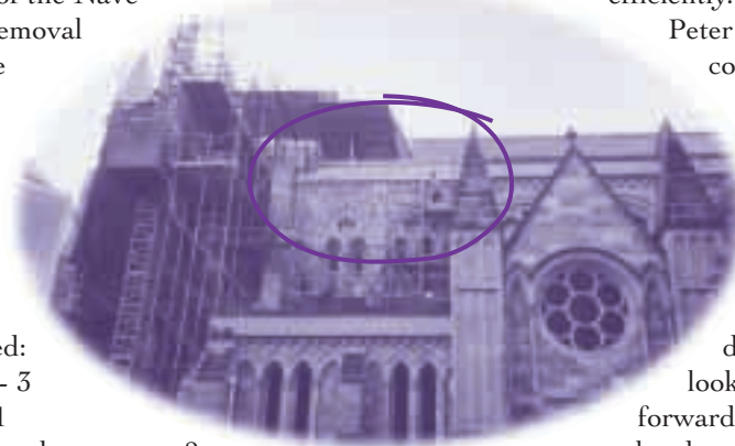
Completed outside Southern Aisle wall
